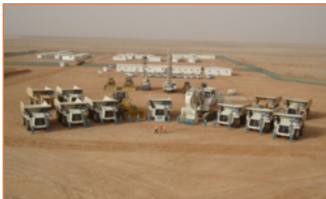
Fleet, accommodation units and key working areas are all tagged.
